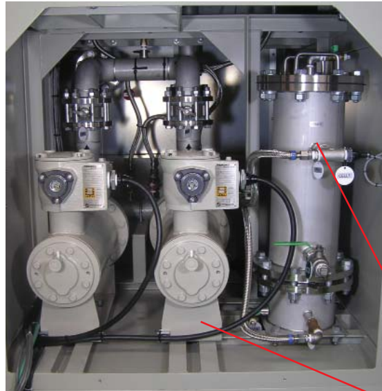
Water conditioning system behind Gate Drive Panel
